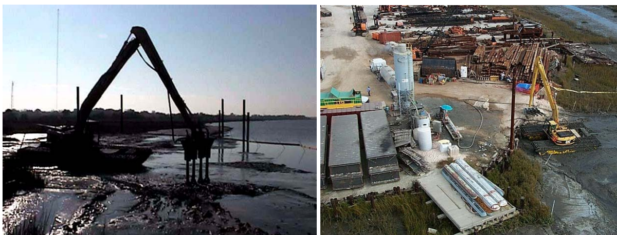
Figure A-9. Rake injector (left) and grout plant and rake injector (right) for treating contaminated sediment at Koppers Co., Inc. (Charleston Plant) Superfund Site, Charleston, S.C. Source: Williams Environmental Services, Inc.
