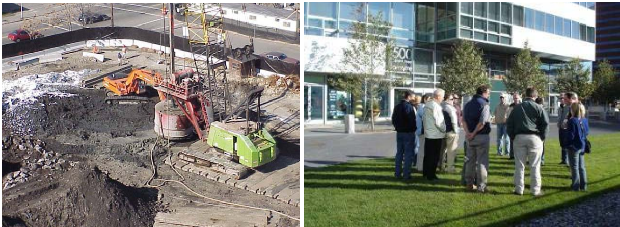
Figure 8-2. Auger-mixed in situ S/S treatment of a former MGP site at Kendall Square, Cambridge, Massachusetts (left) and after redevelopment (right). Source: Portland Cement Association; Carleo, Clark, and Wilk 2006.
