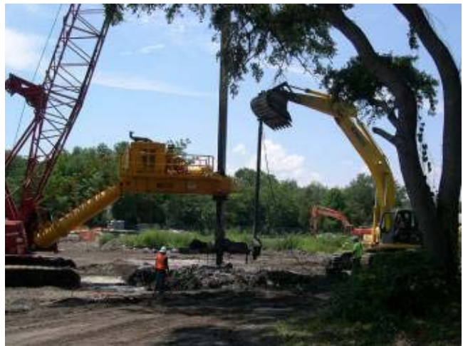
Figure 6-3. Specialized sampler for S/S column mix areas. Source: Ed Bates.
