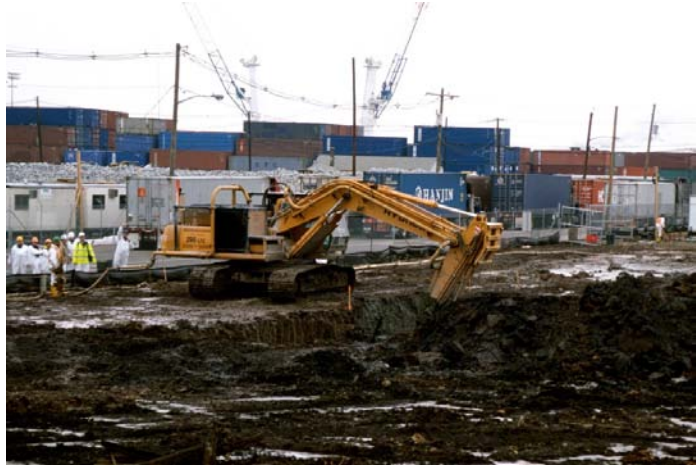
Figure A-1. S/S treatment of contaminated soil by rotary blender at former wood-preserving site, Port Newark, N.J. Source: Portland Cement Association.
