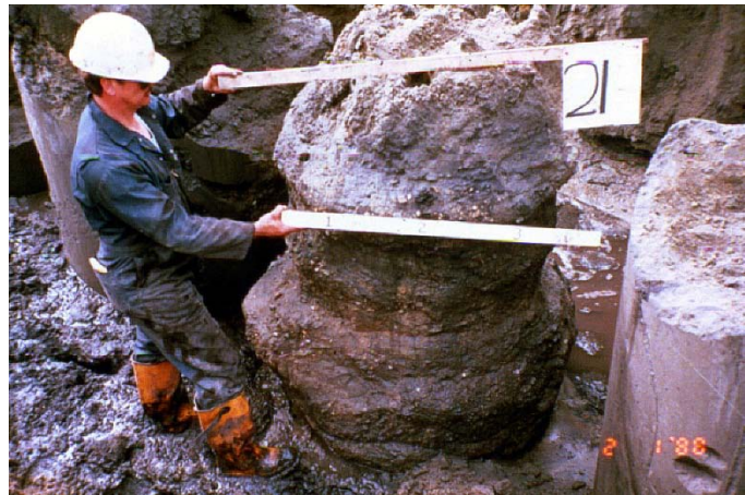
Figure A-13. Exposed jet-grouted columns.
