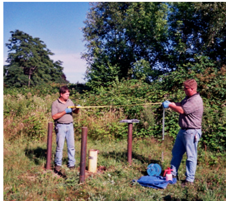
Installation of passive diffusion samplers at the East Multnomah County Cleanup Project
