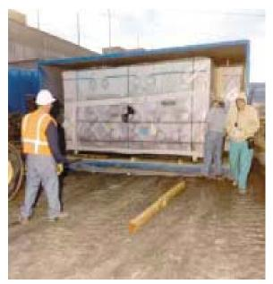
Figure 6-13. After the decontamination process, a glovebox is weighed, packaged, and loaded into a cargo container.
