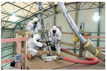
Figure 8-5. Pneumatically removing thorium-bearing waste from Silo 3 at the Fernald Closure Project in October 2005.
