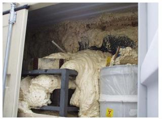
Figure 6-11. Structural foam sprayed into a waste container.
