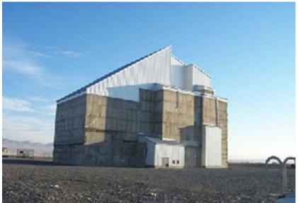
Figure 8-6. Interim Safe Storage (SSE) or cocooning of D Reactor, the fourth of Hanford's nine plutonium reactors to undergo the process, was completed on September 17, 2004.
