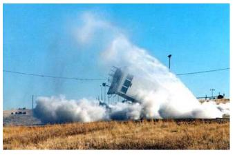
Figure 6-10. Explosive demolition of a guard tower at Rocky Flats.
