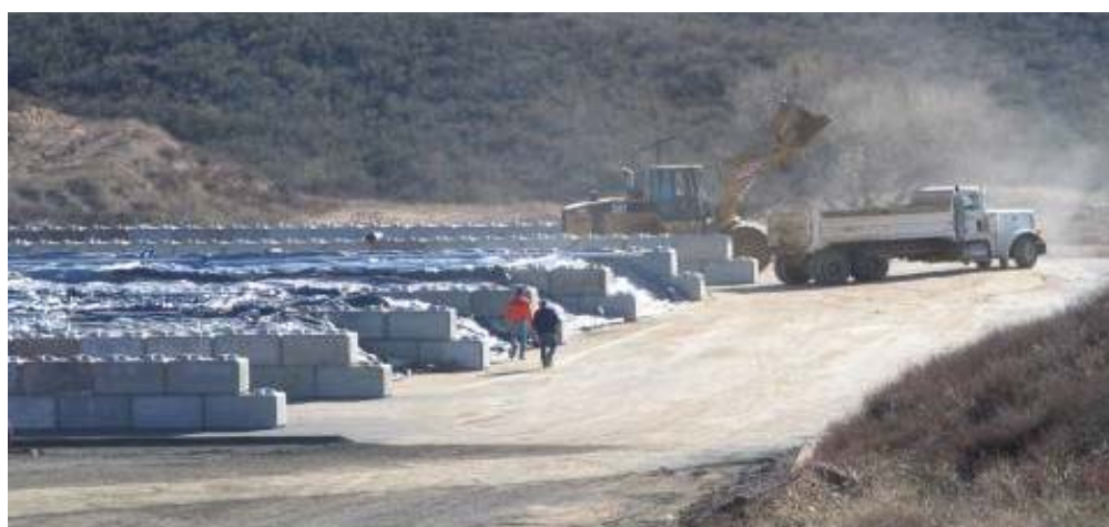
Figure 8-7. Cement-lined treatment cells. (Courtesy CDM Corp.)
