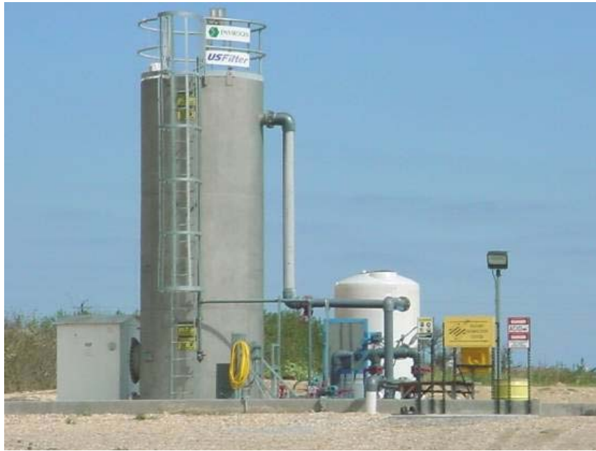
Figure A-37. FBR installed at Area M.
