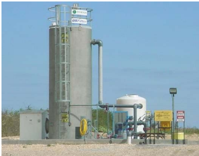
Figure 7-4. McGregor Naval Weapons Industrial Reserve Plant FBR.
