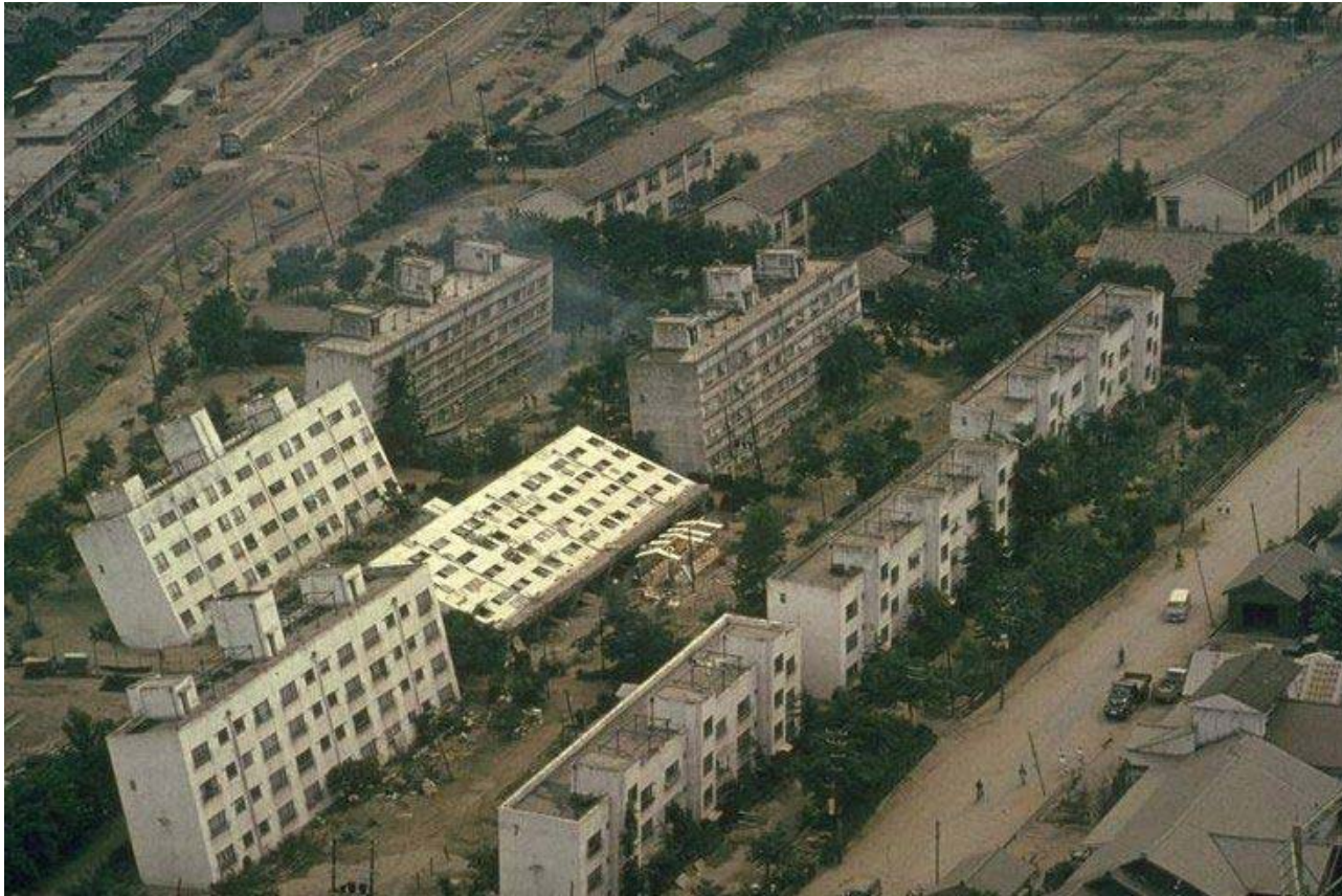
1964 Earthquake – Niigata, Japan
